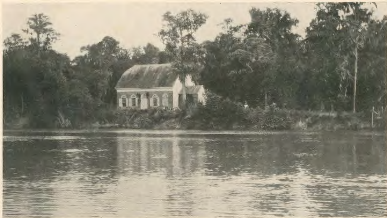
POMPION HILL CHAPEL Eastern Branch Cooper River. Built, 1763.
