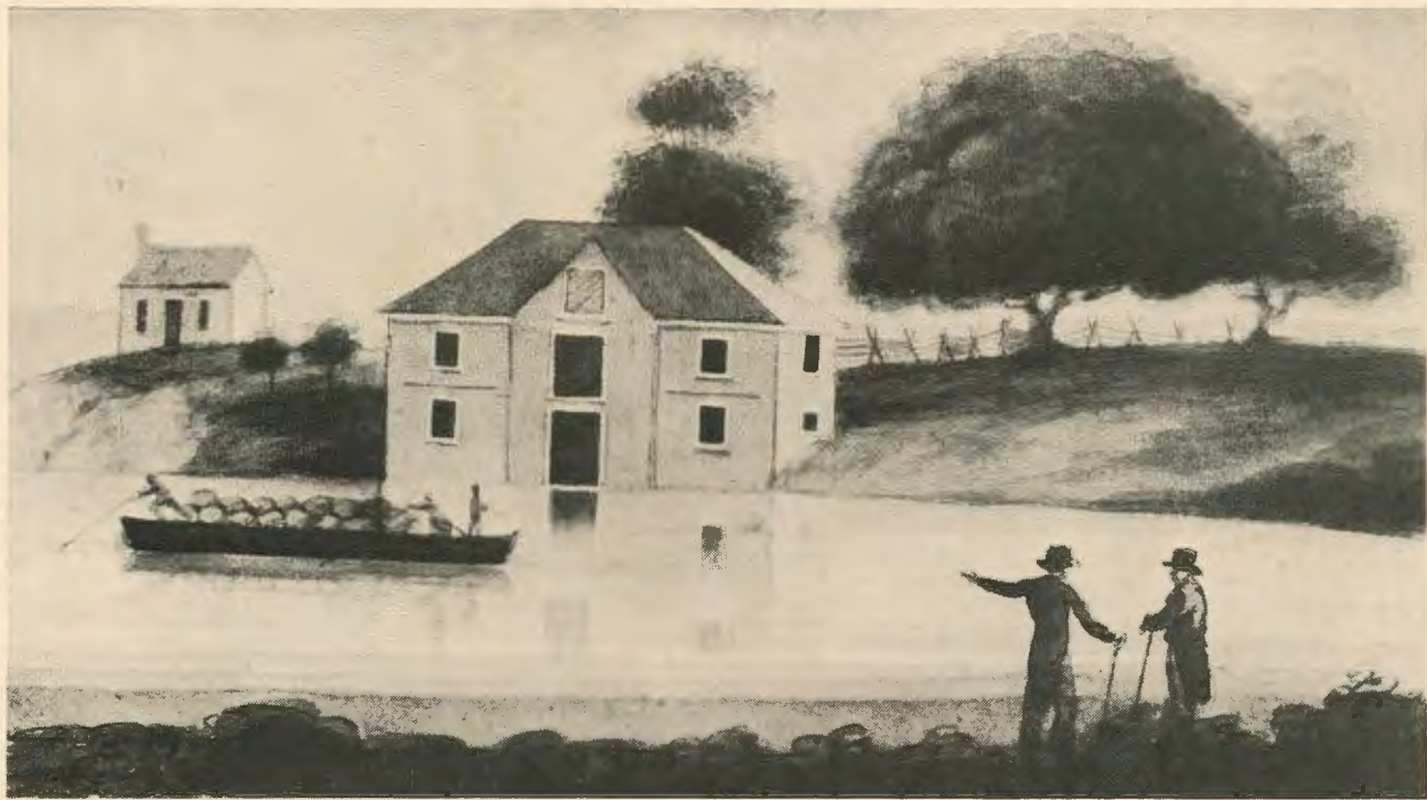
SIMPSON'S BASIN AND STOREHOUSE OLD SANTEE CANAL, 1803
